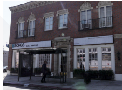
The western portion of Sunset Boulevard features many examples of historic commercial architecture
