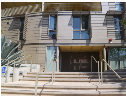
Permanent supportive housing with LEED Platinum rating for sustainability.
