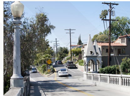
Built in 1926, the Shakespeare bridge provides a whimsical connection between Franklin Hills and Los Feliz
