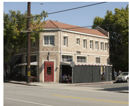
Many older properties in Hollywood required seismic retrofitting after the 1994 Northridge Earthquake
