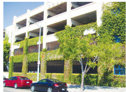
Screening above ground parking lots with greenery makes for a more pleasant walking experience
