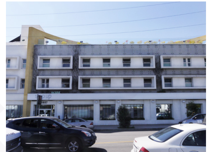
Rehabilitated buildings like Step Up on Vine provide much needed housing and services for the homeless
