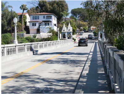
Trees, bridges, lamp posts, and landscaping all add important historical context to neighborhoods
